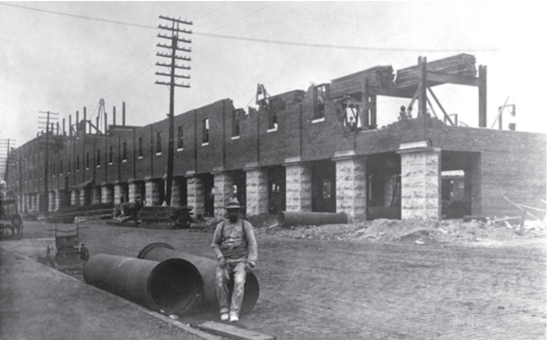
Longworth Hall under construction // all construction photos from www.longworthhall.com/about
